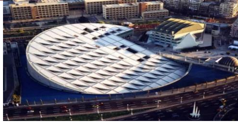
Figure.21. Egypt Library of Alexandria
